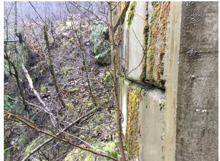
Lock blocks on DS right approach starting to push out on 2nd and 3rd rows
