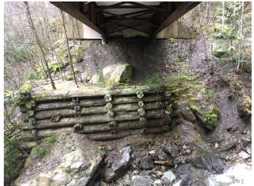
Right Bank Abutment when facing downstream
