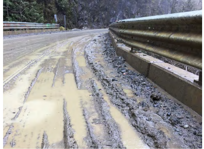
Amount of sediment on deck
