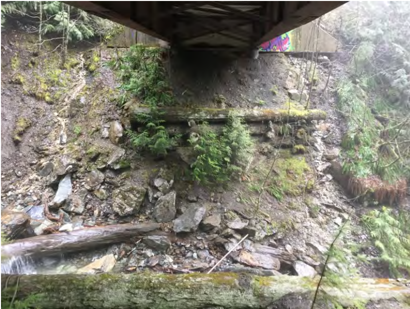
Left Bank Abutment when facing downstream
