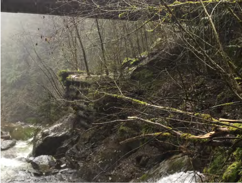
Old log crib left in place right bank - for fill retention check record drawings
