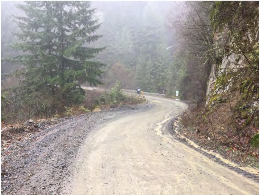
Approach from Left Bank when facing downstream
