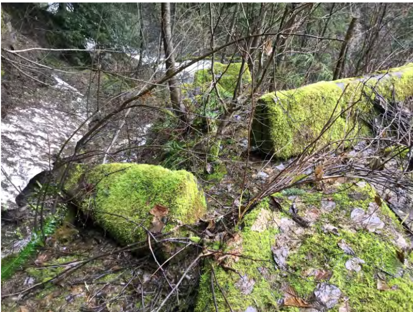
Upstream right approach detached bullnose
