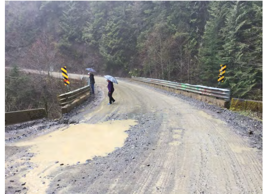
Approach from Left Bank when facing downstream
